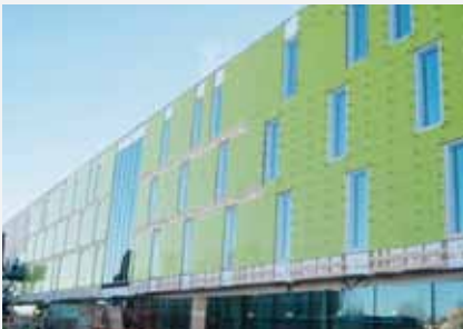
Scandic Oslo Airport, Gardemoen. Entreprenör: Skanska.
